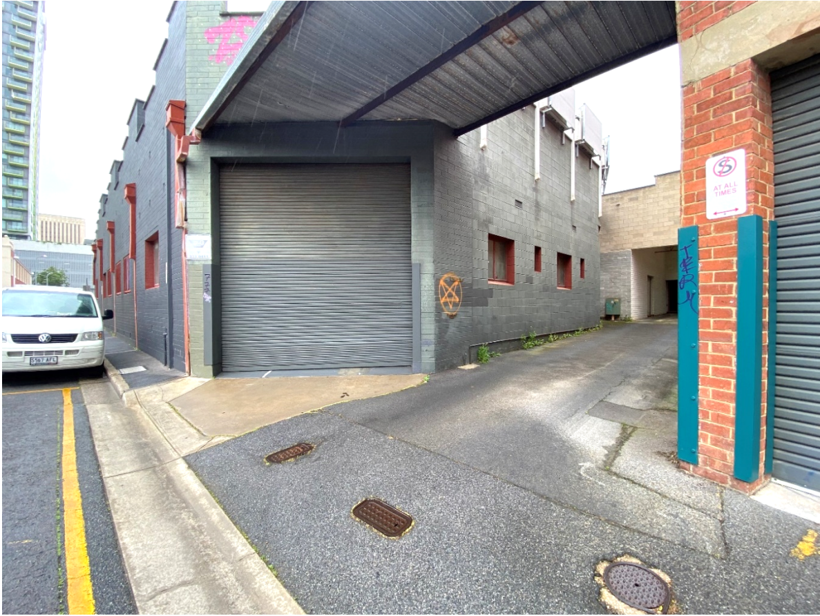
Figure 2.3 - Right of way and rear of the subject building
