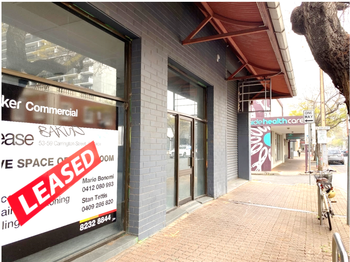
Figure 2.2 – Subject site viewed from Carrington Street looking west
