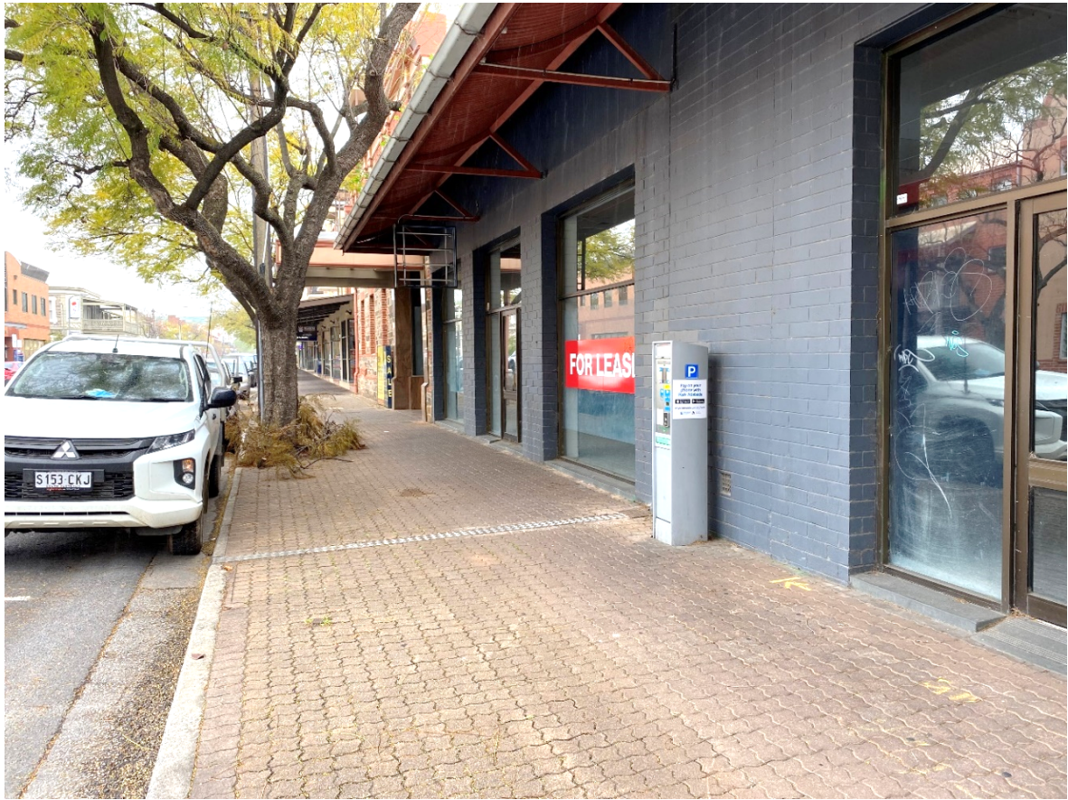
Figure 2.1 – Subject site viewed from Carrington Street looking east
